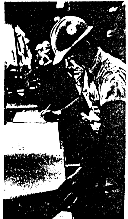
In the Missile Site Control Building, Gary, Washburn County, N.D., checked over plans for the structure described by the Army as, in some respects, the "last of its kind ever to be built" ▶
