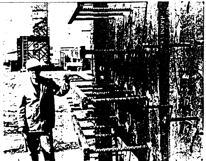
LEO CARDENAS, ASSOCIATED with the Ramsey Steel firm of El Paso, Texas, which manufactured the steel tubes, stands beside one of the cans being prepared for emplacement. The anchor bolts are embedded in concrete. The plate at side is over two inches thick and weighs more than 800 pounds. Architectural engineering for the "cans" was a tricky business never before done.
