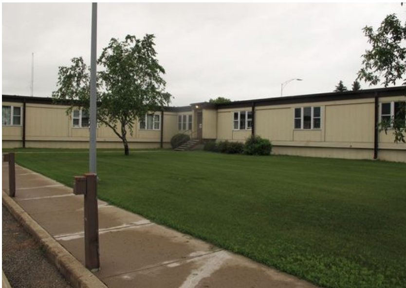
A dormitory on the Cavalier Air Force Station built as a temporary housing structure and was described by one base captain as an "elongated trailer house." (Photo: Dave Kolpack/AP)
