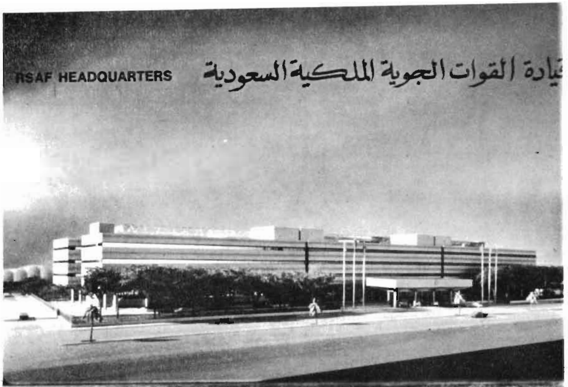
Royal Saudi Air Force Headquarters (RSAF) as constructed by the Corps.
