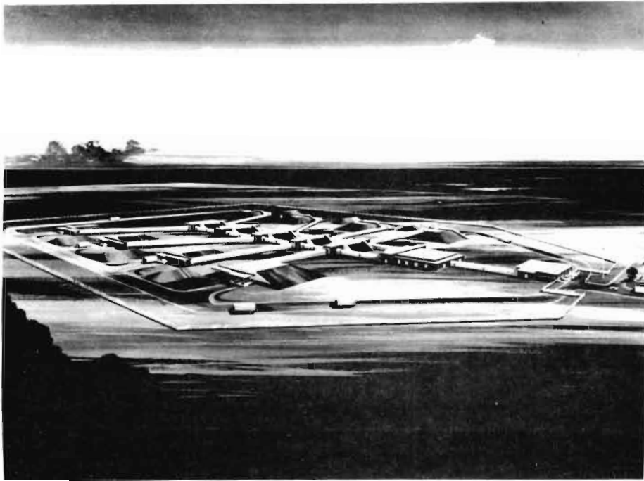
Central X-Ray Facility, Milan, Tennessee
