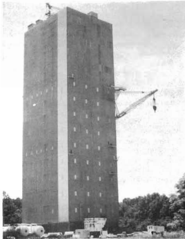
"SPACE SHUTTLE MATED GROUND VIBRATION TEST FACILITY" (Building 4450 Marshal Test Center) converted for Space Shuttle Testing.
