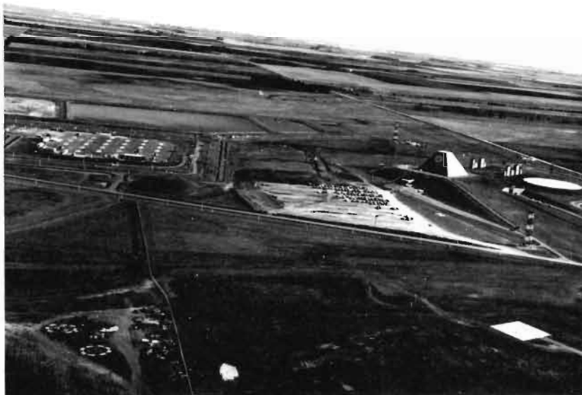
TACTICAL FACILITIES OF THE SAFEGUARD BALLISTIC MISSILE DEFENSE SYSTEMS' MISSILE SITE RADAR site constructed near Grand Forks, North Dakota. Right foreground is the Helipad; right is the circular underground heat sink; to its left the intake and exhaust stacks of the underground power plant; the turret of the partially buried Missile Site Control Building; to the left the Spartan and Sprint Missile Fields; and the mounded earth covered Missile Assembly Building.
