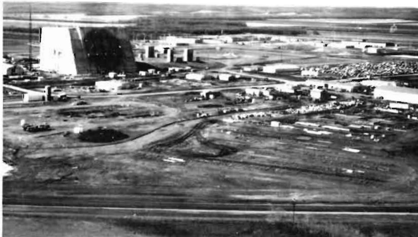
PAR FACILITIES of the SAFEGUARD Ballistic Missile Defense near Grand Forks, North Dakota, as they appeared on April 19, 1972. At the upper left is the PAR control building with its associated power plant to the right. In the background are some of the support facilities of the installation. In the center and on the right are temporary contractor buildings and workers' automobiles.
