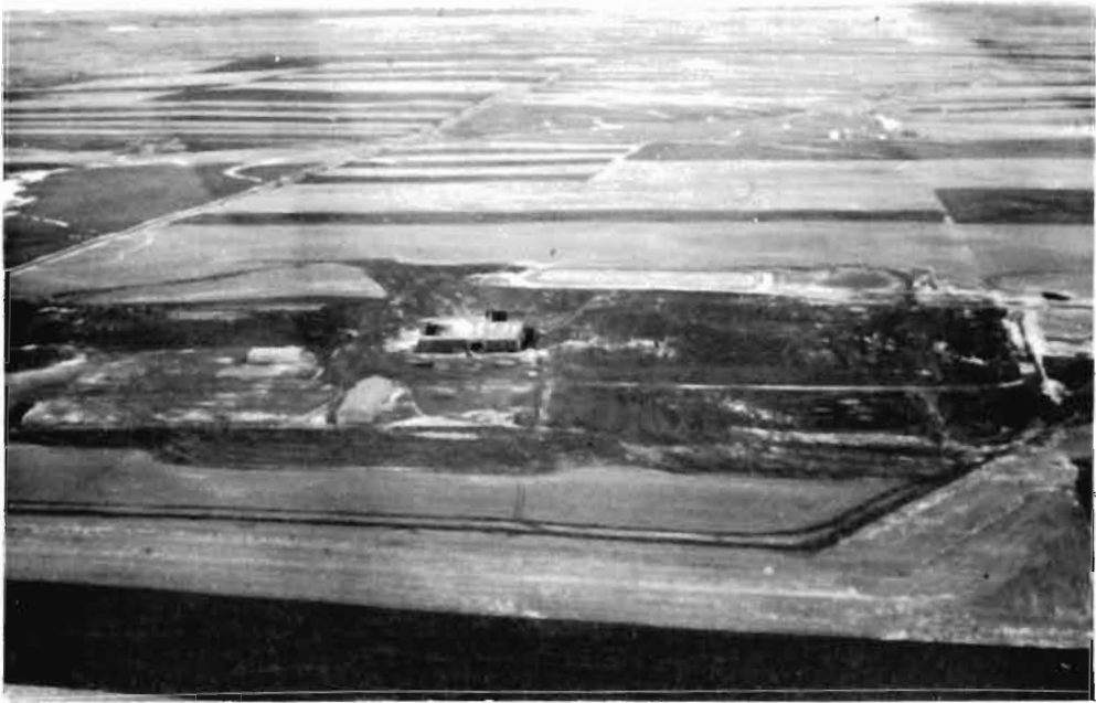
MALMSTROM PAR SITE after restoration work. Buildings were donated to local government agencies. (May 1974)
