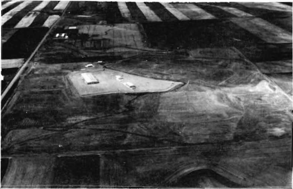
MONTANA MSR SITE after restoration (May 1974) Building left were donated to local government agencies.
