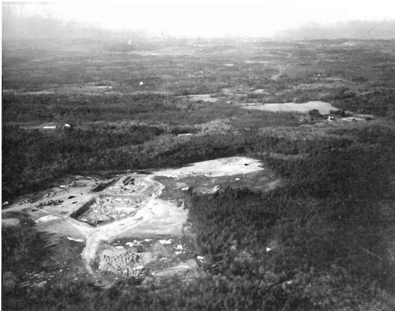
SHARPNER'S POND AFTER SUSPENSION OF WORK, MARCH 1970
