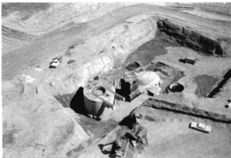
Launch Facility under construction in the mid-1960s.
