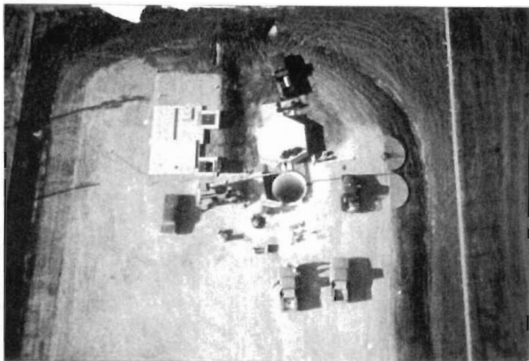
Launch Facility at Grand Forks, under construction.
