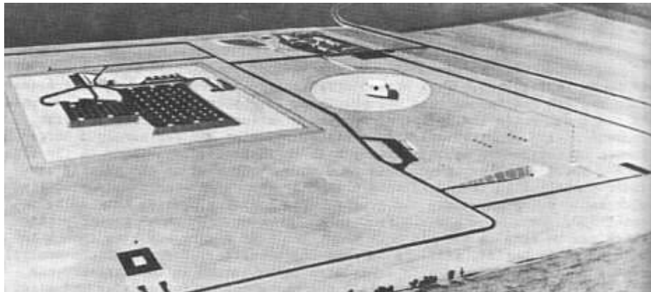
Figure 4. Missile Site Radar Installation
