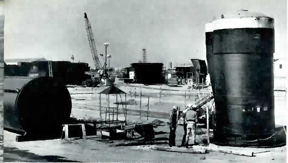
ABOVE, LEFT, steel shell for 31-foot-deep silo to house Sprint missile is prepared for installation in shaft; RIGHT, mechanical gear is moved into PAR building.
