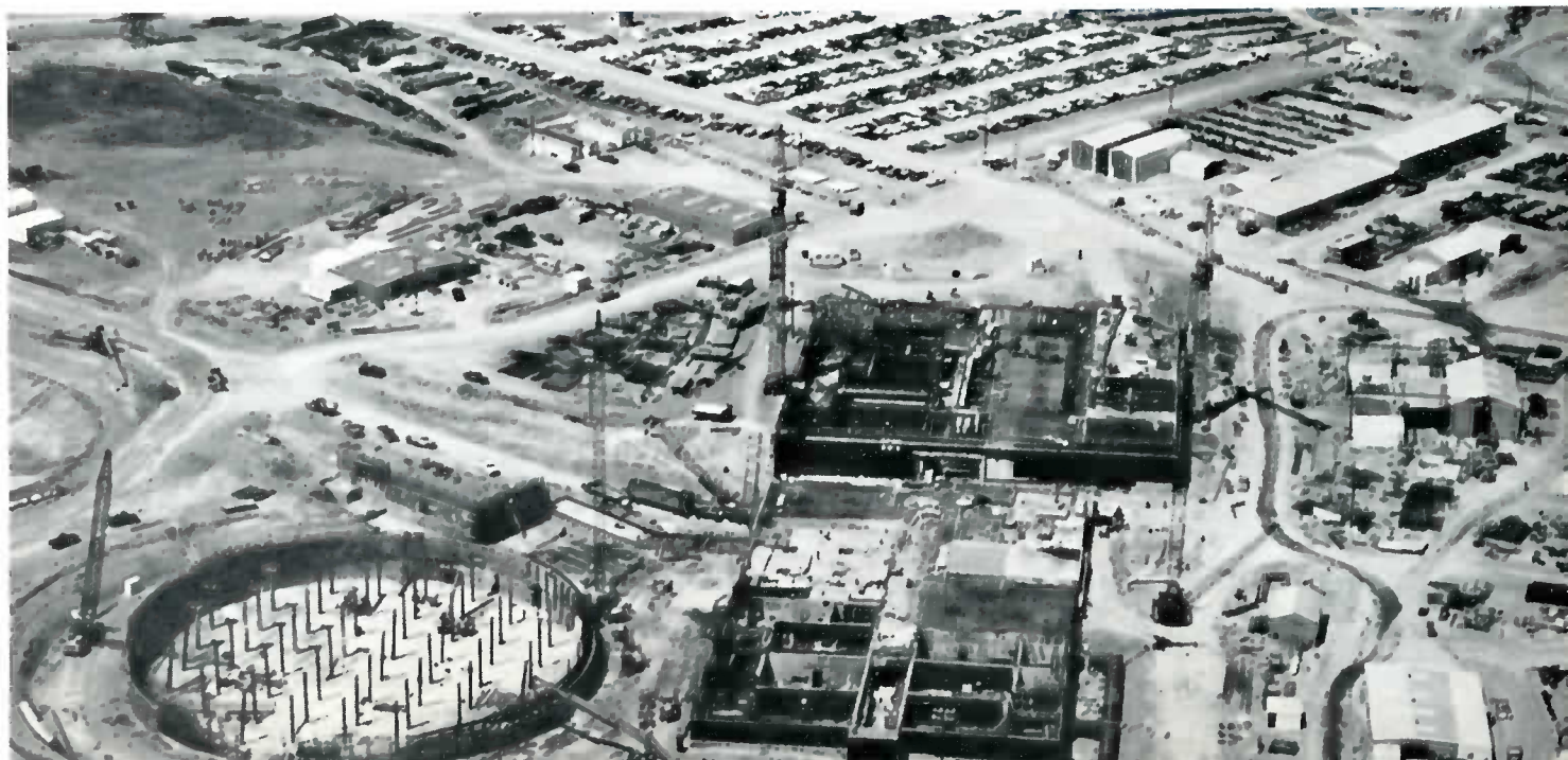
ABOVE, LEFT, sketch of Missile Site Control Building, with 78-foot-high turret atop structure reaching 48 feet beneath surface; RIGHT, sketch of 125-foot-high PAR building, with long-range antenna on north wall. BELOW, aerial view of MSR site shows 7.5-million-gallon heat sink (left), power plant (front) and control building.
