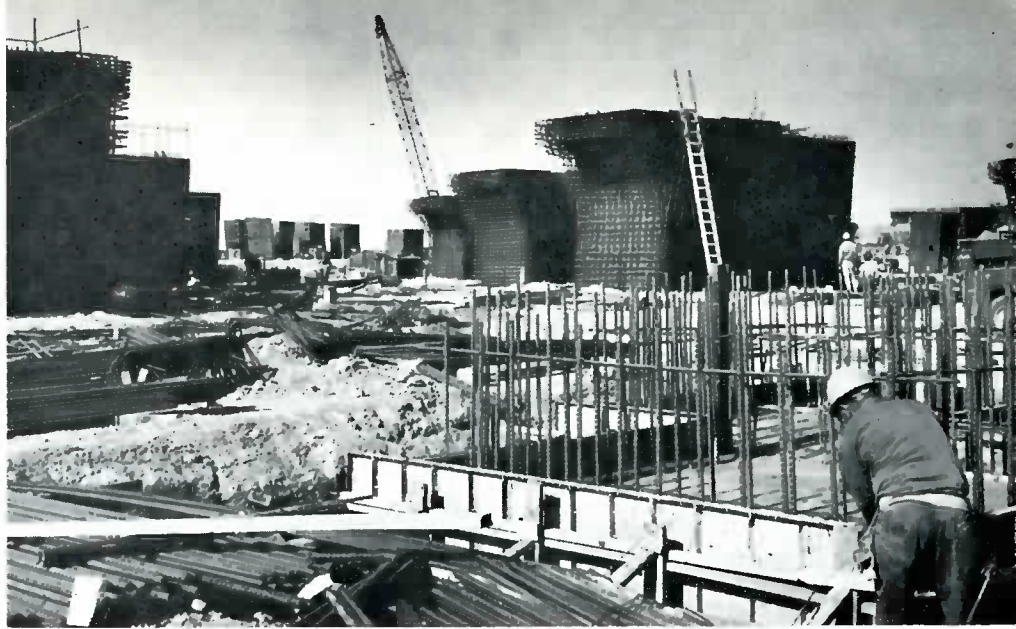
ABOVE, LEFT, fuel and water lines are part of 200,000-foot piping program; RIGHT, wrappings of re-steel near completion on top portions of Spartan missile silos.
